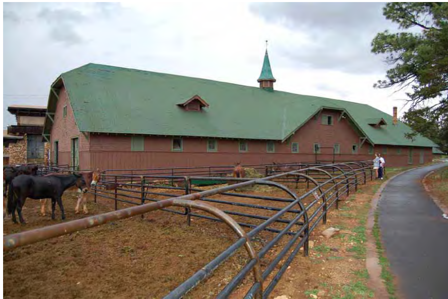
Figure 2 Grand Canyon Village Mule Barn
